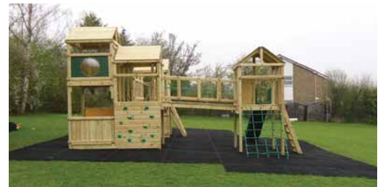
This equipment is arranged in a “L” shape with the Mountain Clubhouses connected to two jungles by bridges.
