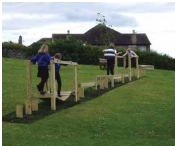
This short play trail has been installed on a slope but each piece has been specially adapted so the equipment is level.
