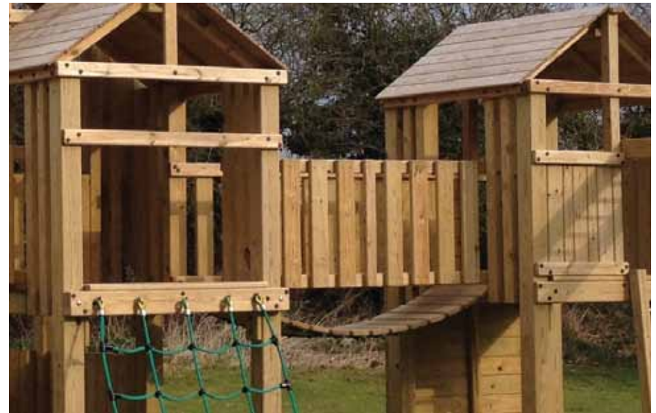
Wobble bridge: deck planks are fixed to steel ropes with small gaps between so the bridge articulates when you cross it.
