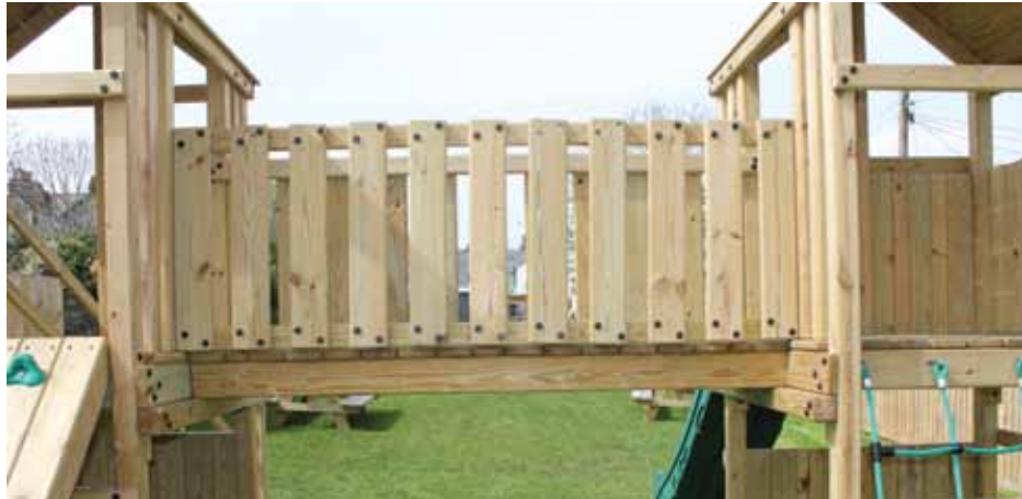
Solid bridge: a rigid deck with planks fixed to solid timber joists.
