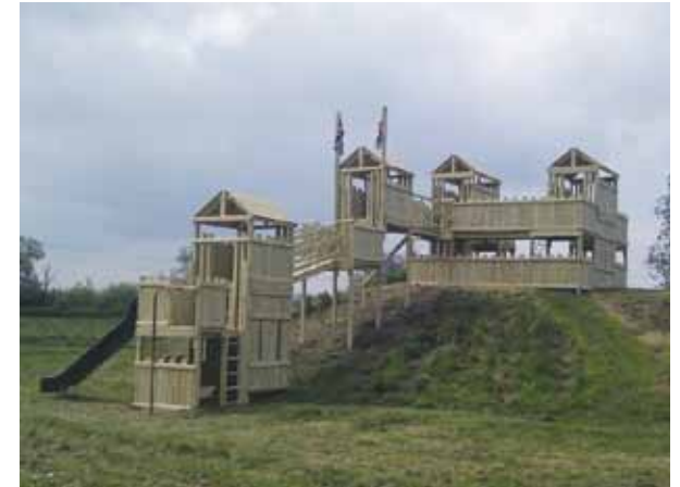
This visitor attraction in the South West wanted a large scale fort but with the severe slope there wasn't enough room on the top; the solution – a series of clubhouses which "cascade" down to base level.
