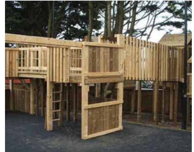
As part of a wider playground development including swings and other climbing equipment, we built a fort which starts in the play area and is linked by bridges to a series of towers in the trees. The bridges were enclosed to keep children in the play zone and lead them back to the main playground.
