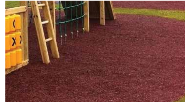
Bonded mulch laid straight onto grass.
