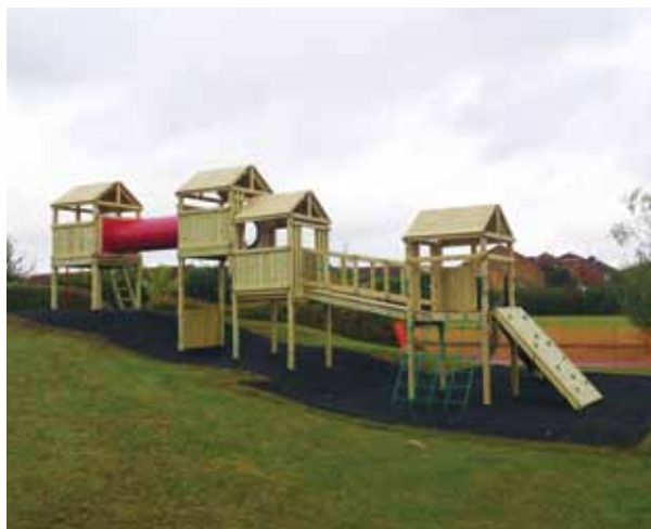
We took advantage of the slope on this school site to have the clubhouses linked to each other with bridges to different deck heights.
